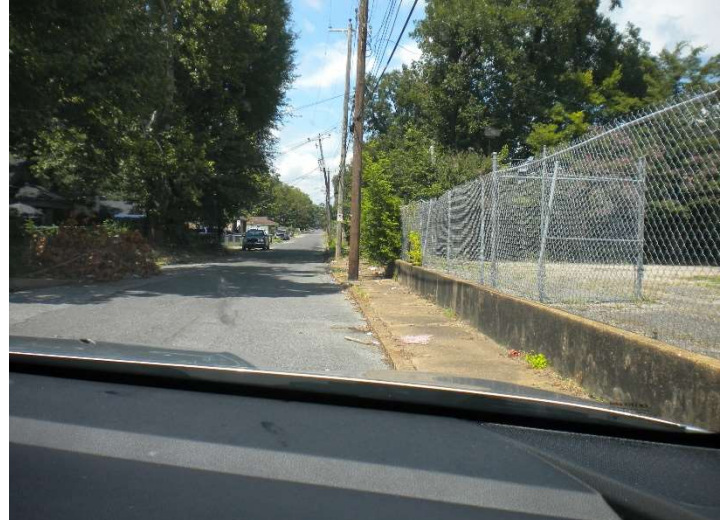
1) Deteriorated street pavement. 2) Narrow and deteriorated sidewalk pavement. 3) Utility poles are not installed within a planting strip, creating a clear path obstruction for pedestrians. 3) Dead and overgrown vegetation obstructs pedestrian access along sidewalks.
