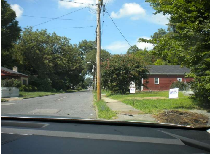
1) Deteriorated street pavement. 2) Deteriorated sidewalk pavement. 3) Overgrown vegetation obstructs pedestrian access along sidewalks.
