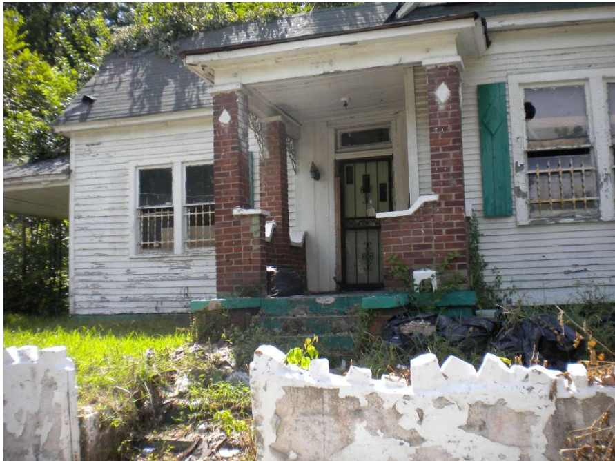
A vacant, deteriorated, single family structure with deteriorated site improvements. Specific conditions include damaged and rotting siding, window framing, roofing, fascia and soffit; broken windows; cracked and crumbling concrete porch and stairs; unmaintained and overgrown vegetation; cracked and crumbling retaining wall; and trash discarded in front lawn.
