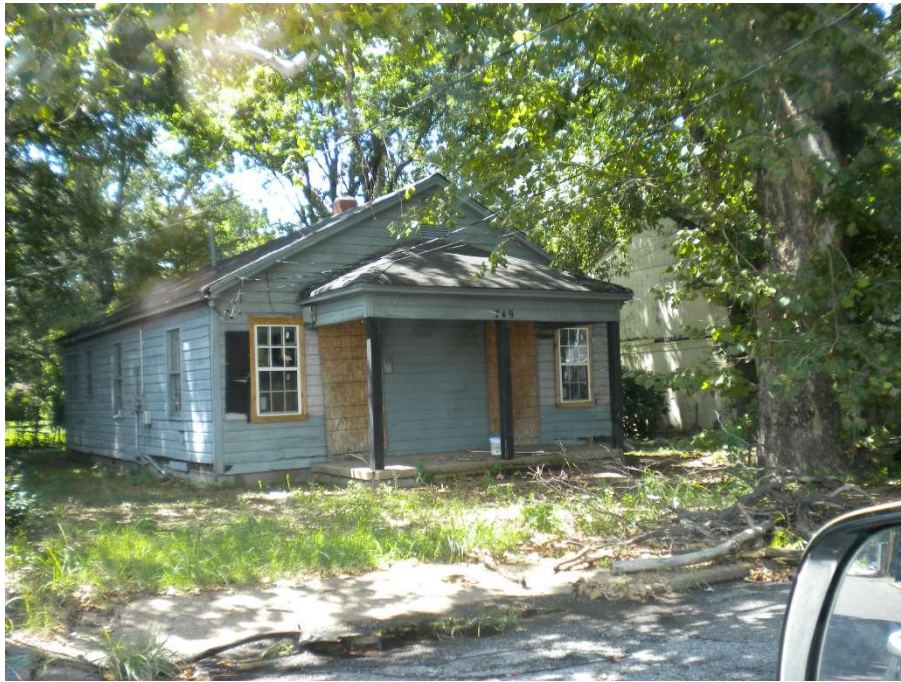
A vacant, deteriorated, two-family structure with deteriorated site improvements. Specific conditions include damage and rotting siding; boarded up front doors; and deteriorated porch and walkway pavement; unmaintained and overgrown vegetation and discard dead tree limbs; deteriorated driveway where curb aprons are constructed.
