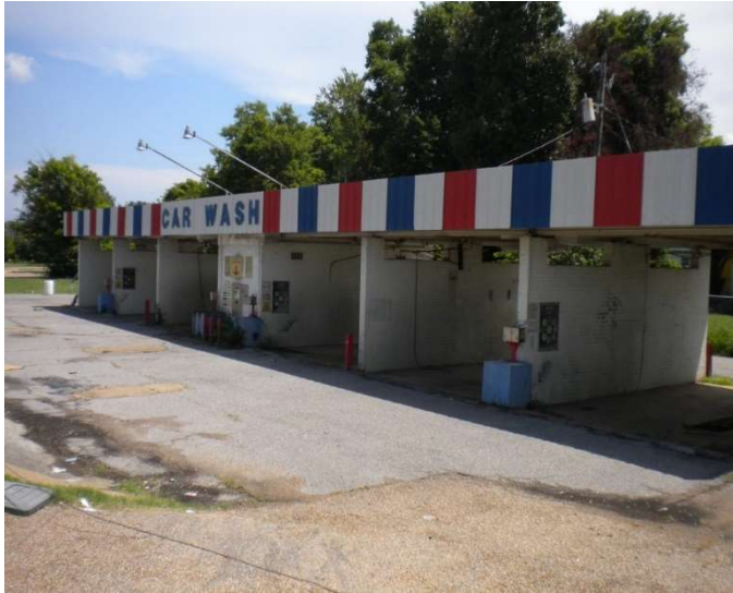
A deteriorated commercial structure with deteriorated site improvements. Specific conditions include deterioration of masonry walls and pavement.
