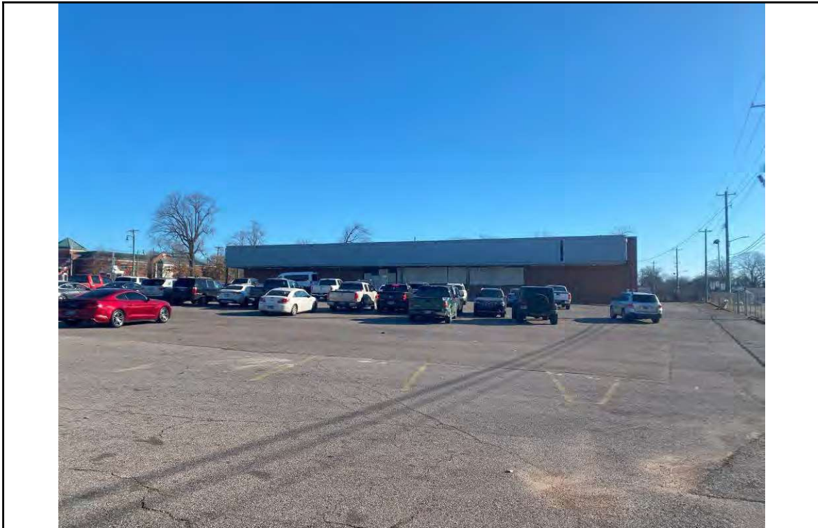
PHOTO NO. 1 DESCRIPTION: View of the asphalt parking lot and the vacant grocery store building on the east portion of the subject property. The parking lot is currently leased to American Lebanese Syrian Associated Charities Inc.
