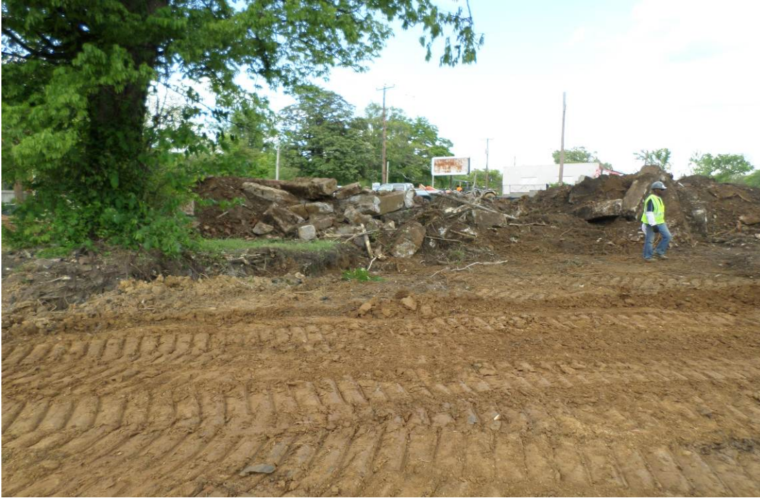
Photo 13: Initial backfill of removal areas with silty clay.
