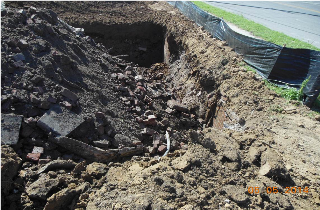
Photo 9: Continued debris removal from Basement #2.
