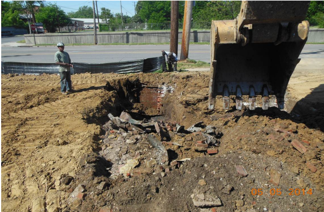
Photo 7: Continued debris removal from Basement #2.
