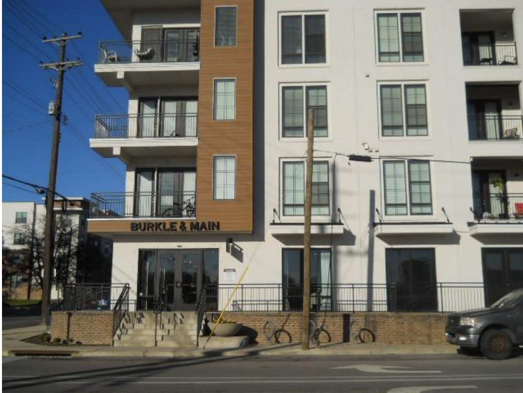
Photo #23 View from the site looking north across Chelsea Avenue towards Burkle & Main located at 800 North 2 nd Street
