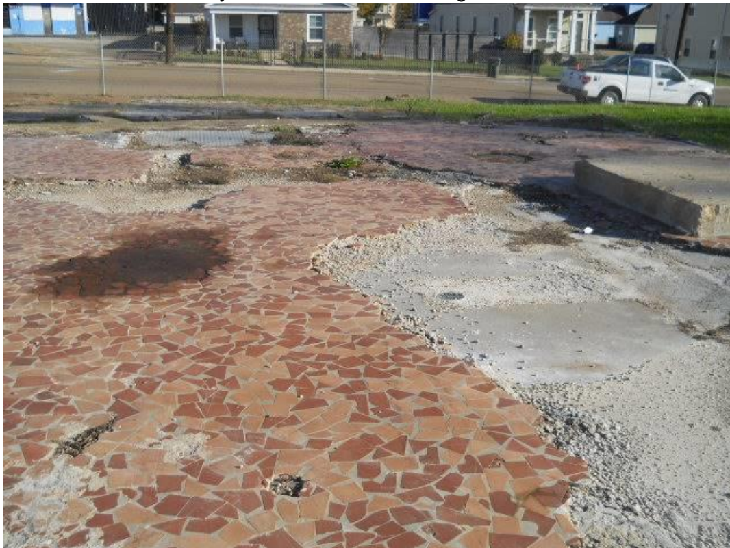
Photo #36 View of de minimis staining on the ceramic flooring
