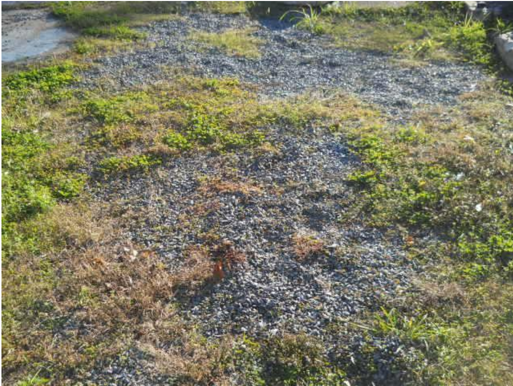
Photo #43 View of gravel area east of the former Wayne's Pinball Palace foundation
