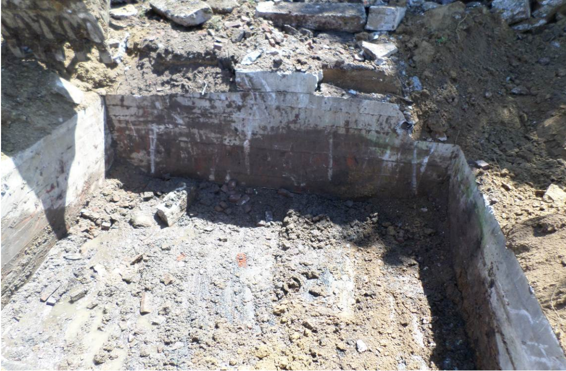
Photo 5: Basement#1 is cleared before removal of walls and floor.
