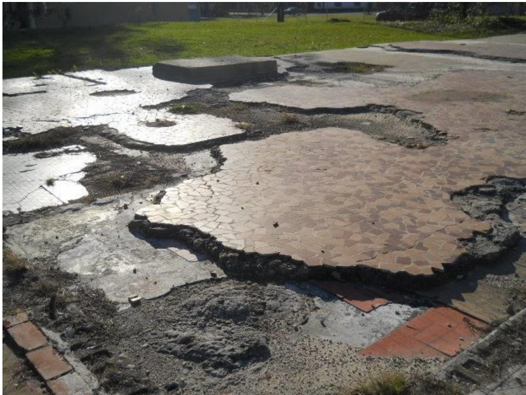
Photo #42 View of assorted flooring located below ceramic flooring layer
