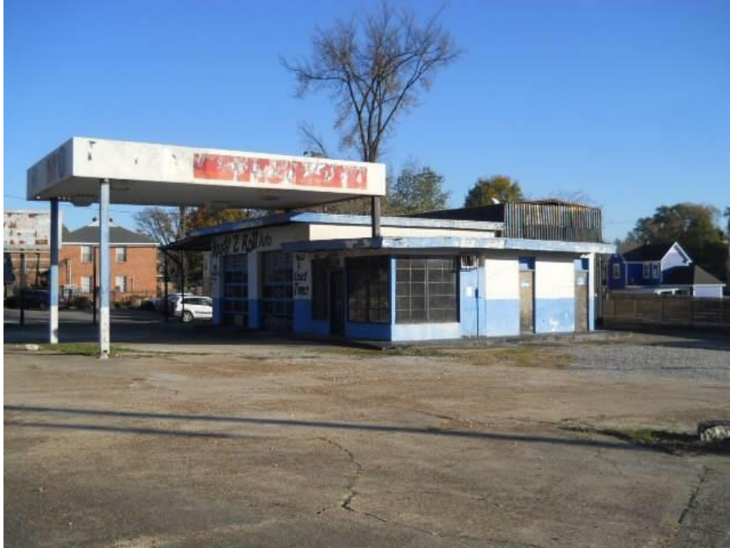
Photo #21 View of former Ready 2 Roll located at 183 North 3 rd Street
