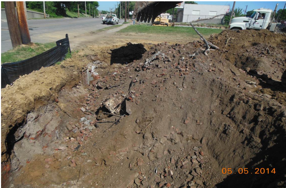
Photo 8: Continued debris removal from Basement #2.
