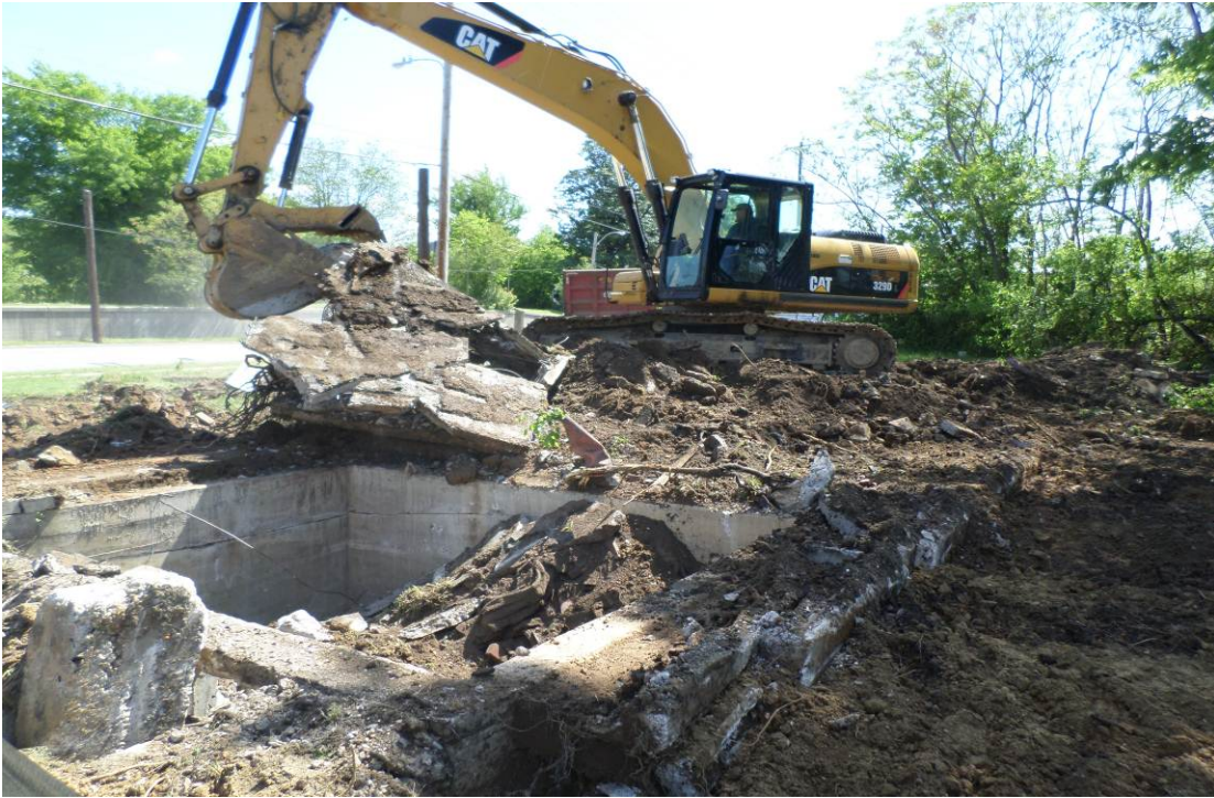
Photo 3: Removal of top of Basement#1.
