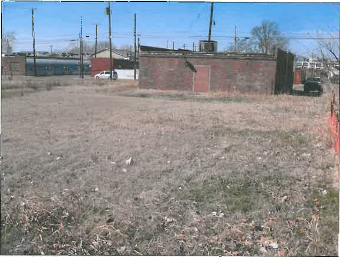
Photo 5: Typical view of the exterior of the subject property facing west.
