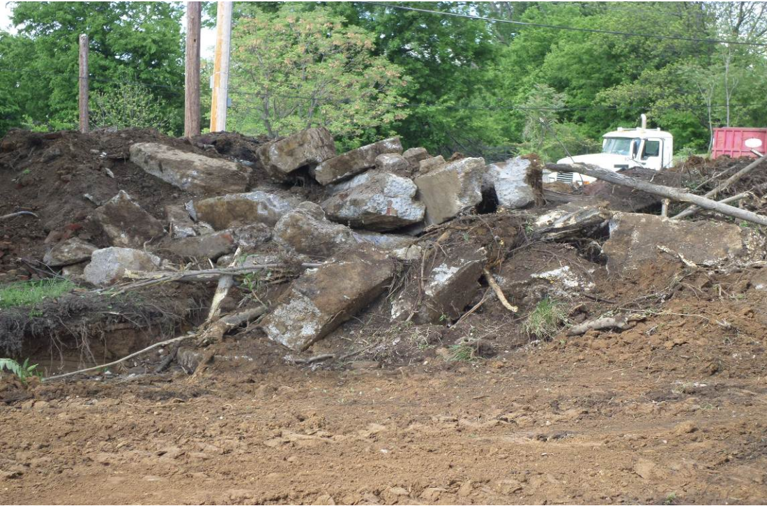
Photo 11: Stockpiled concrete debris from foundations that were previously onsite.
