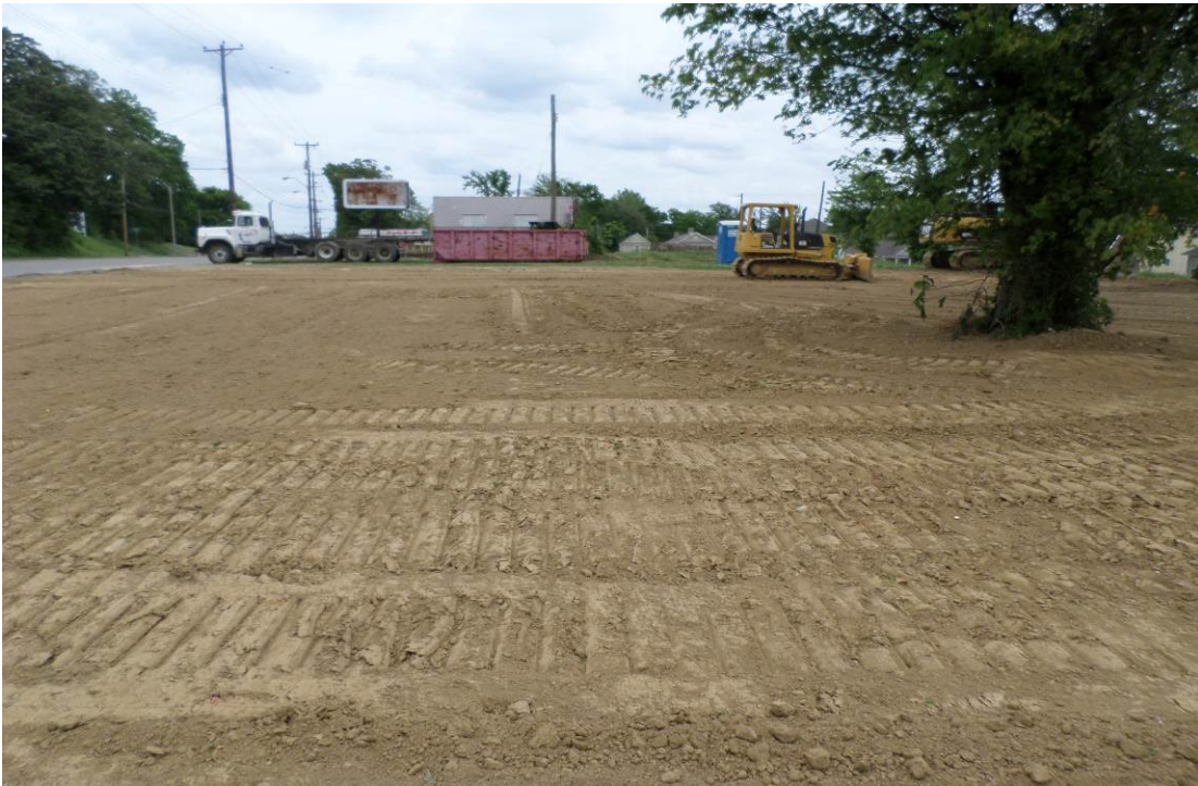
Photo 14: Final grading and backfill of basement removal areas with silt clay.
