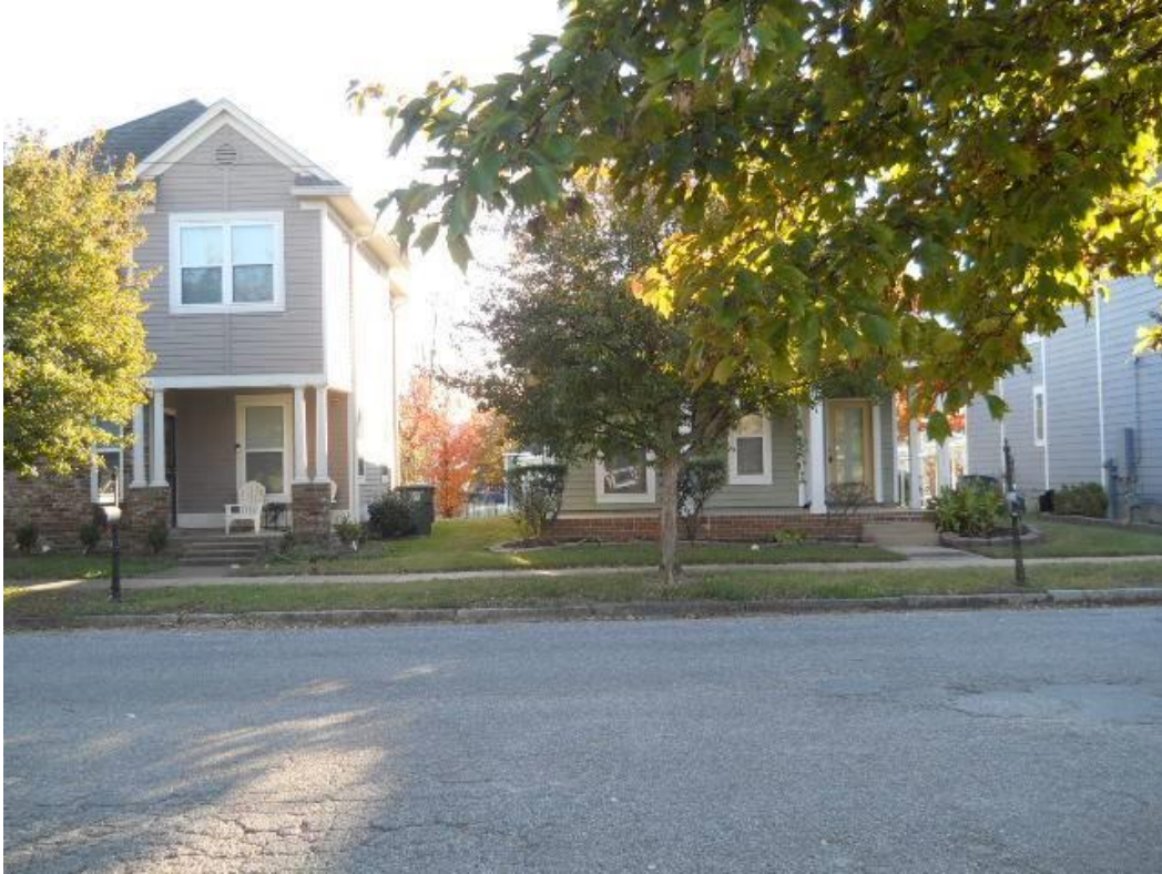
Photo #29 View from the site looking south across Keel Avenue towards south-adjointing residences
