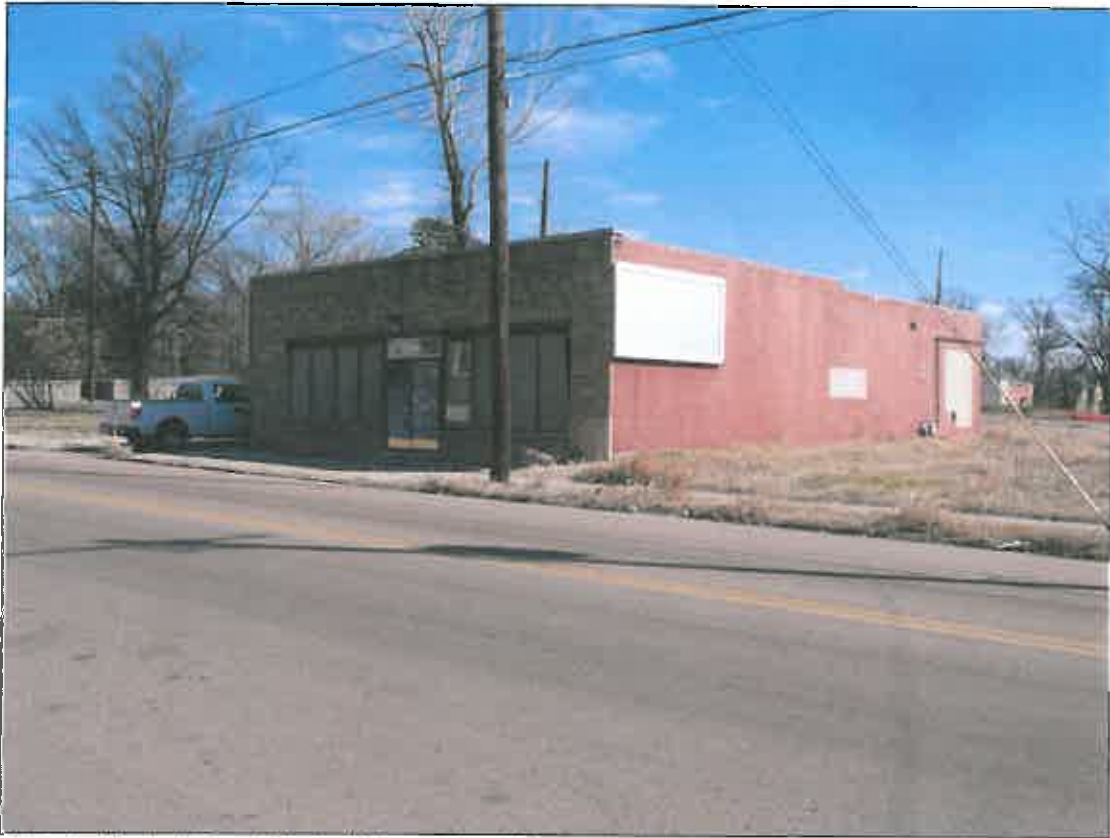
Photo 1: Typical view of the building on the subject property.
