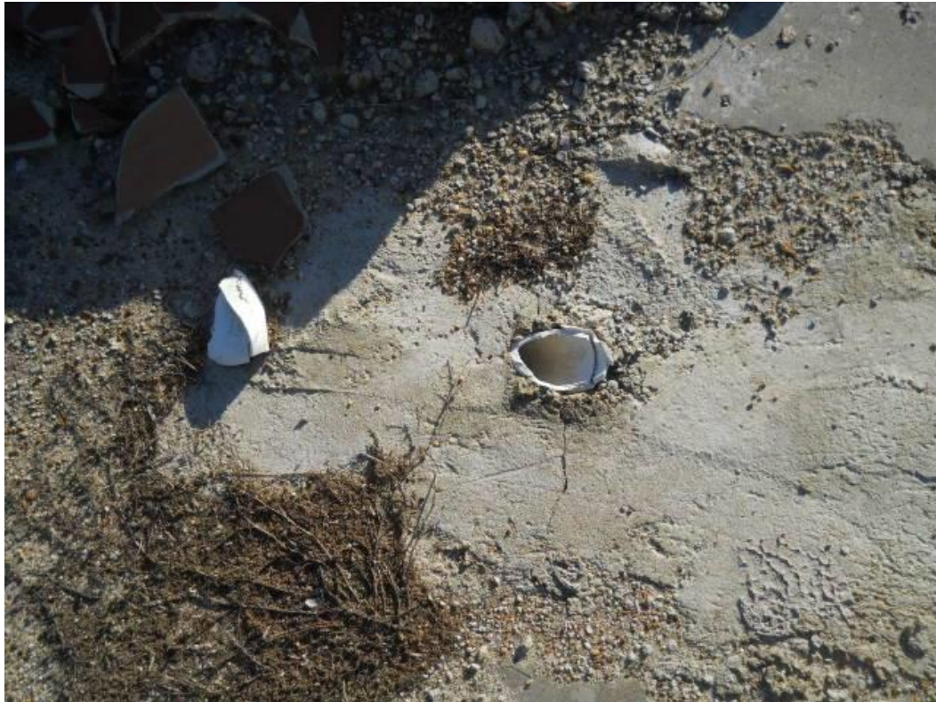
Photo #41 View of a PVC pipe located in the concrete foundation
