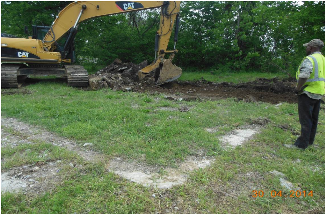
Photo 1: Initial clearing of underground concrete structures.
