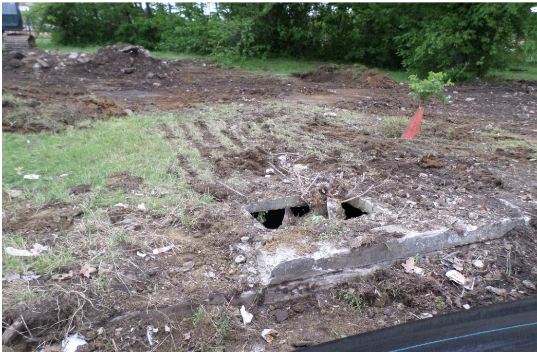
Photo 2: Initial surface clearing of topsoil above Basement #1.
