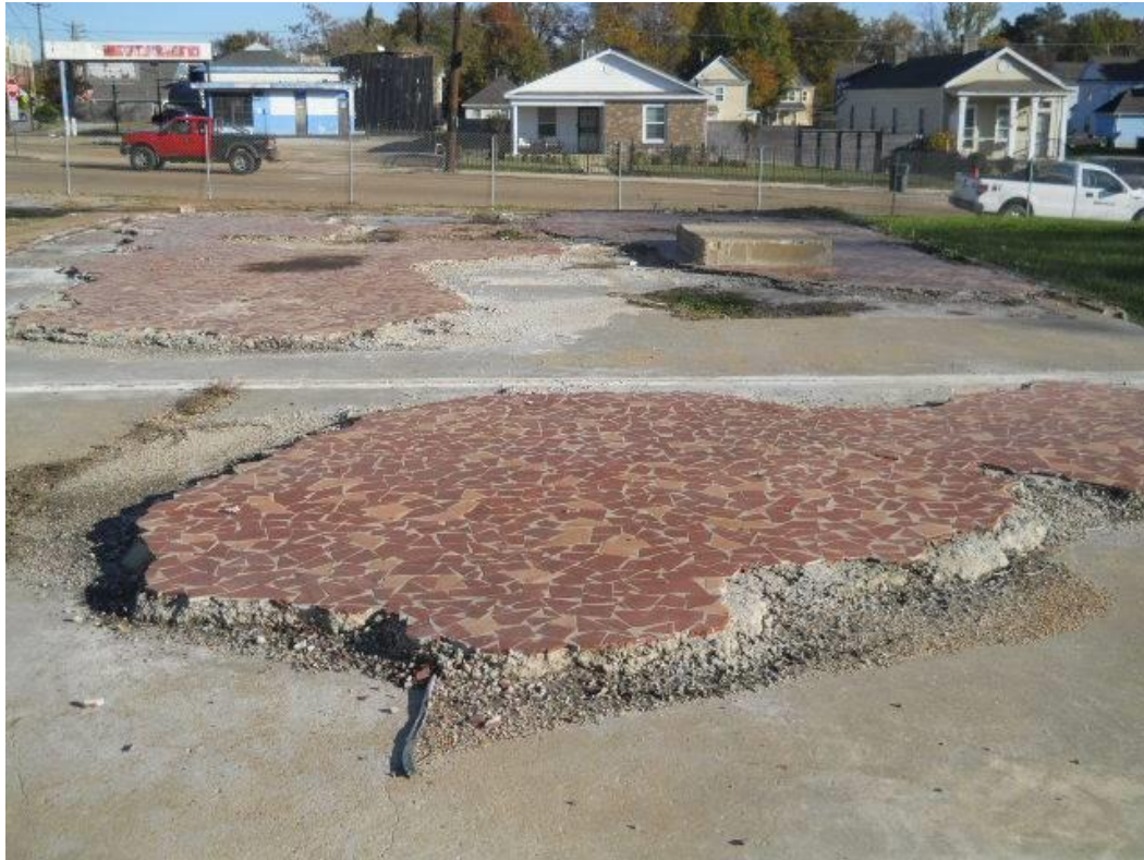
Photo #35 View of concrete foundation and old flooring located on the northeast block of the site where the former Wayne's Pinball Palace existing
