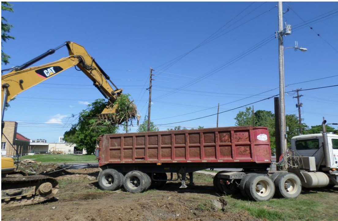
Photo 12: Loading of C&D debris (trees) before transport to the landfill.
